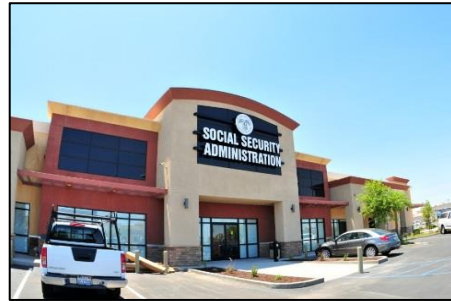
$8,500,000 Social Security Office El Centro, California Status: Funded
